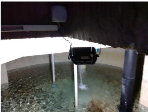
Blick in Schacht
